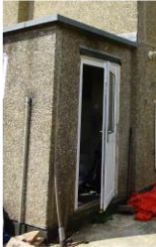
S61 – 31 Victory Road, Whiteshill. Side extension view from rear
