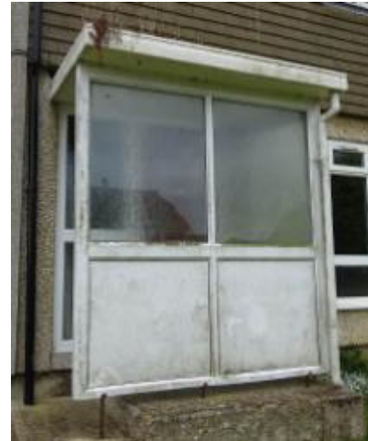
Q8 – Typical front porch without door
