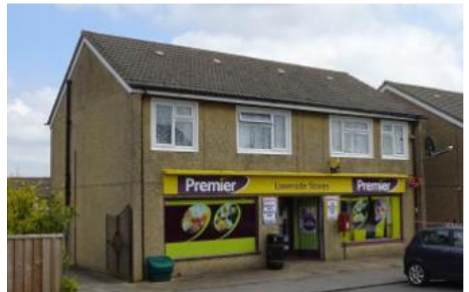
S14 – Flat & Shop in Lawnside, Forest Green
