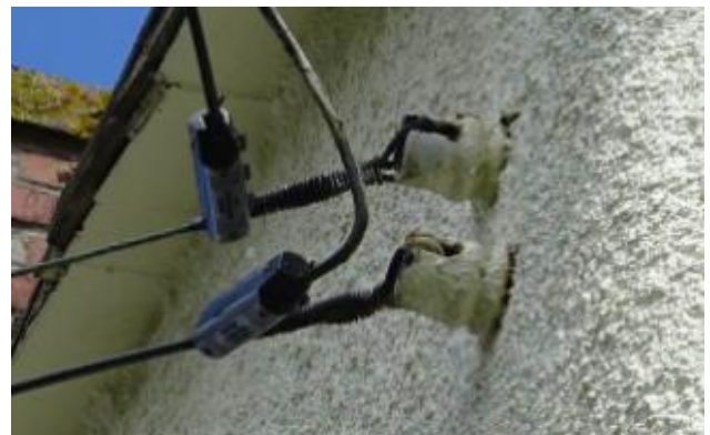
P10 – Overhead power supply fixing at wall, at 10 Kingley Road, Cashes Green
