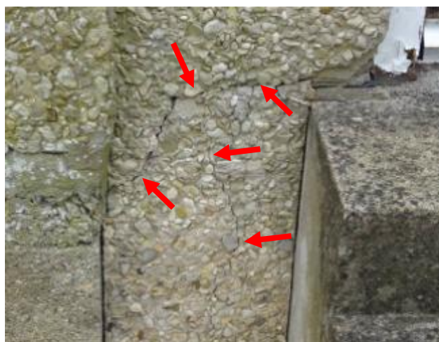
S41 – 6 Upper Park Road, Nailsworth. Cracking at dpc to side of door
