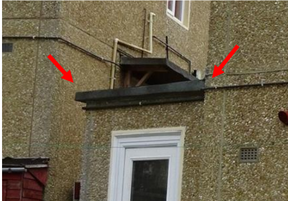
S55 – 5 Upper Park Road, Nailsworth. Flat roof side extension (compare with S39, lean-to roof No 6)
