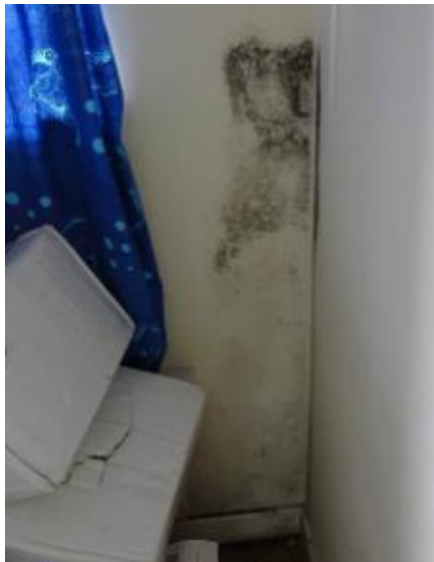
S21 – 12A Lawnside, Forest Green, Bedroom mould to right of window mid height
