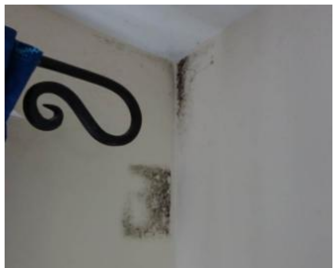
S18 – 12A Lawnside, Forest Green, Bedroom mould to right of window high level
