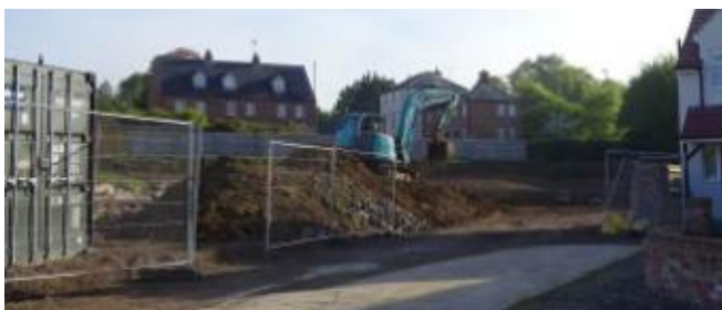
S15 – Site at Wharfedale Way, Bridgend, two Reema houses demolished (Nos 8 & 10)
