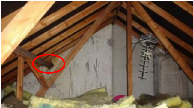
S51 – 3 Upper Park Road, Nailsworth. General View in Loft towards the party wall (S52 circled)
