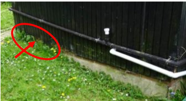
T9 – 32 Barrs Lane, North Nibley. Outbuilding side, ground level too high (circled). Rot to outer boards at dpc level (T10 circled)
