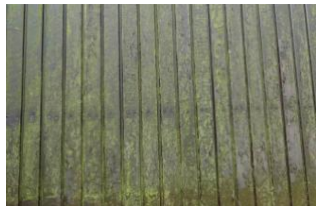
T18 – 3 Bushey Beeches, The Camp. Side elevation, algae growth on outer boards
